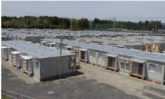
Temporary housing complex for victims of the Noto Peninsula Earthquake (April 2024)
