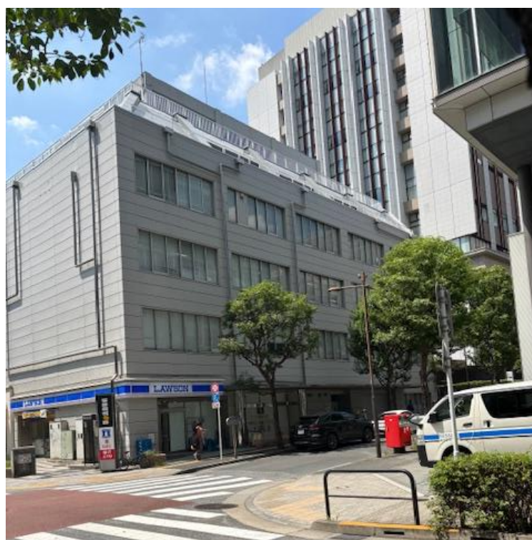
The NTT Surugadai Building, Chiyoda-ku, Tokyo, where the BHN Headquarters Office is located after the relocation
