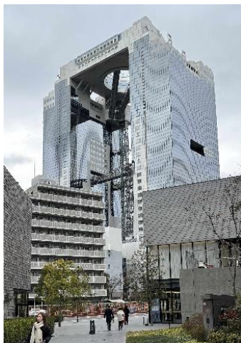
The Umeda Sky Building in Osaka as an exhibition venue
