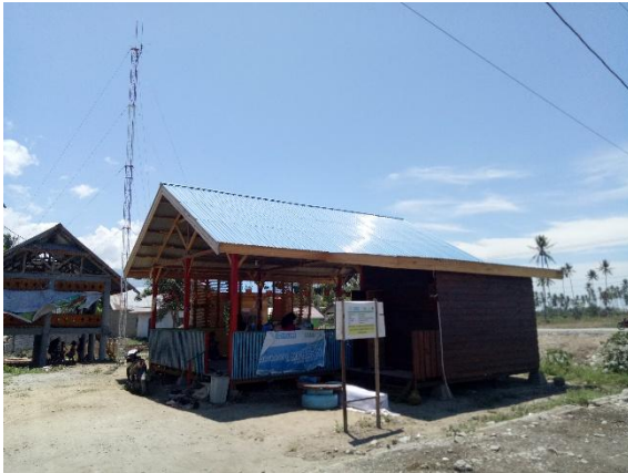
Photo A-2 Community radio station building and antenna tower
